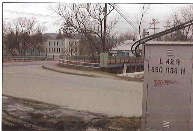
LOOKING FROM SOUTH TO EAST
