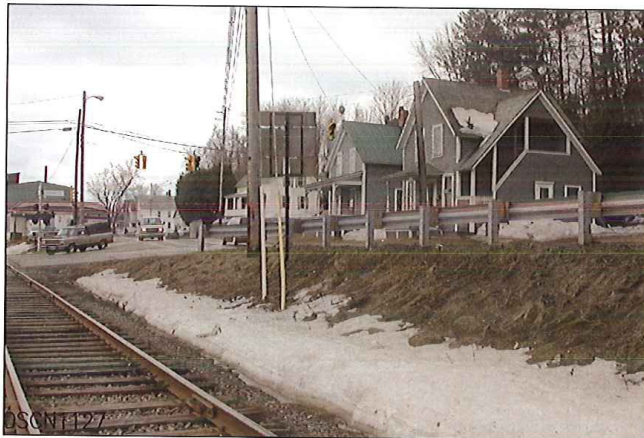
LOOKING FROM NORTH TO WEST
