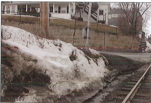
LOOKING FROM SOUTH TO WEST
