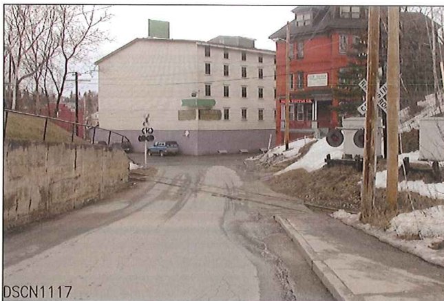
LOOKING FROM WEST TO EAST
