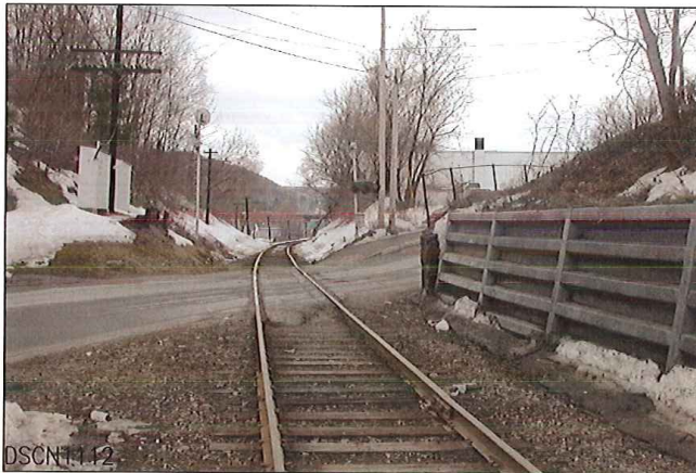
LOOKING FROM NORTH TO WEST
