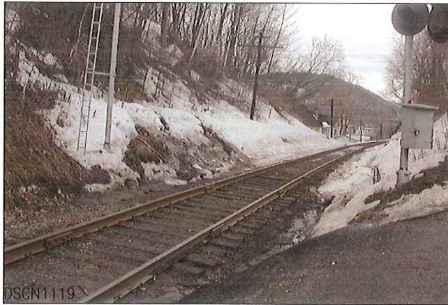
LOOKING FROM WEST TO SOUTH
