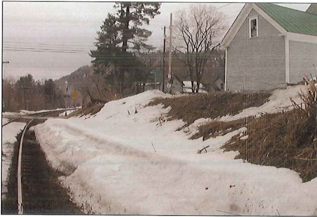
LOOKING FROM NORTH TO WEST
