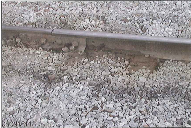
SOUTH RAIL, EAST OF CROSSING
