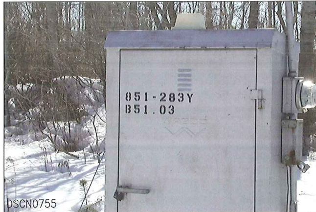
SOUTH EAST QUADRANT
