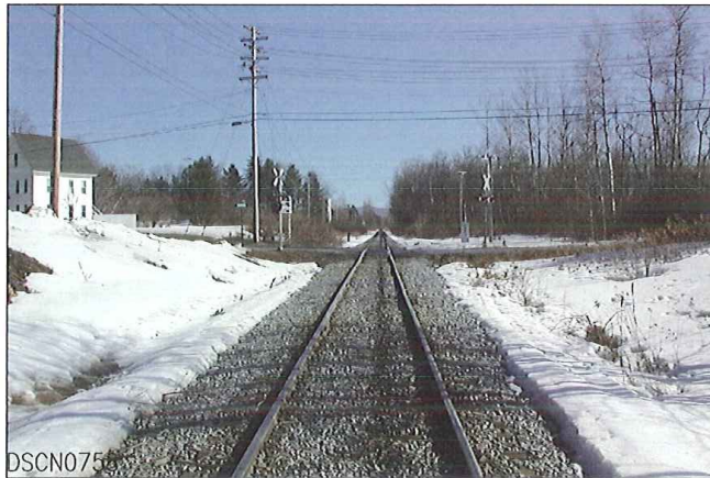
LOOKING FROM WEST TO EAST
