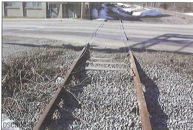
ABANDONED SIDETRACKS SOUTH OF MAINLINE
