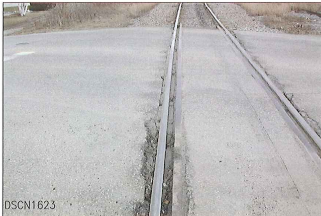
LOOKING FROM WEST TO EAST
