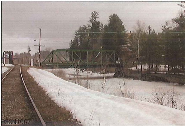
LOOKING FROM SOUTH TO EAST
