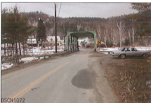
LOOKING FROM WEST TO EAST
