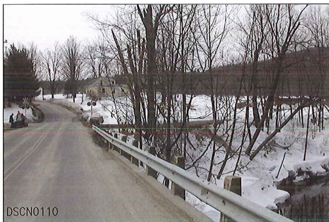
LOOKING FROM NORTH TO WEST
