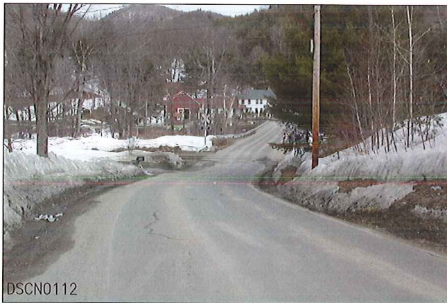
LOOKING FROM SOUTH TO NORTH
