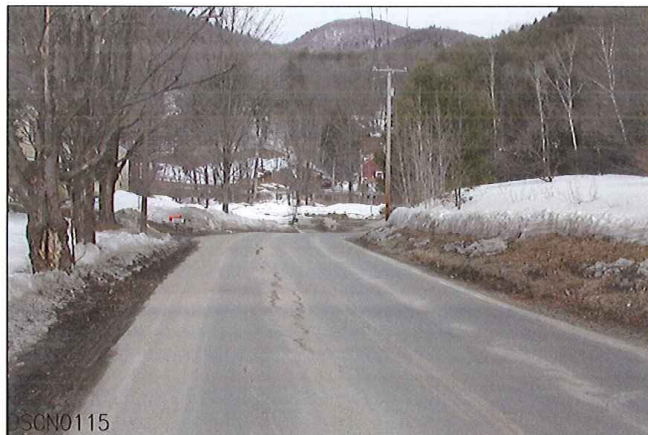
LOOKING FROM SOUTH TO NORTH
