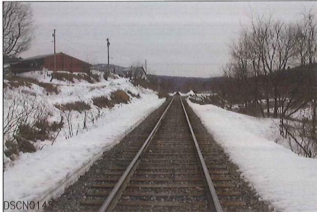
LOOKING FROM WEST TO EAST
