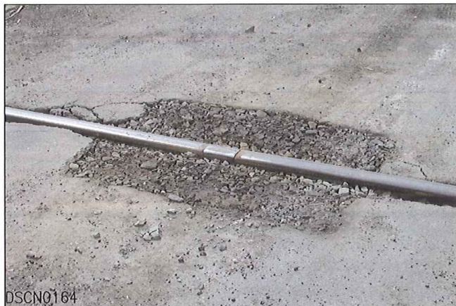
SOUTH RAIL — DUTCHMAN INSTALLED
