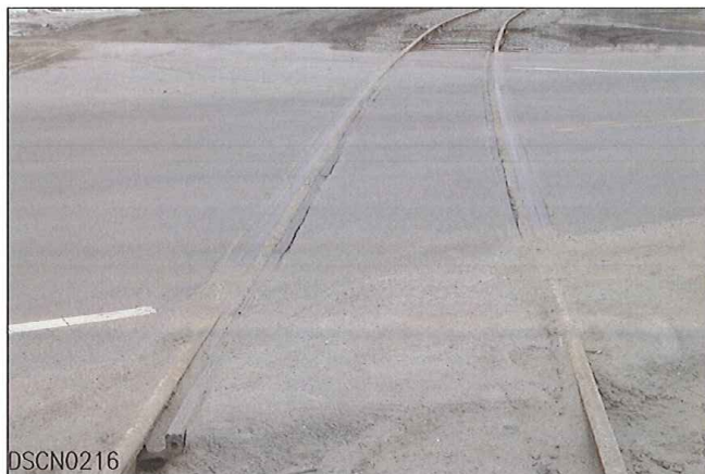
SIDE TRACK LOOKING FROM EAST TO WEST
