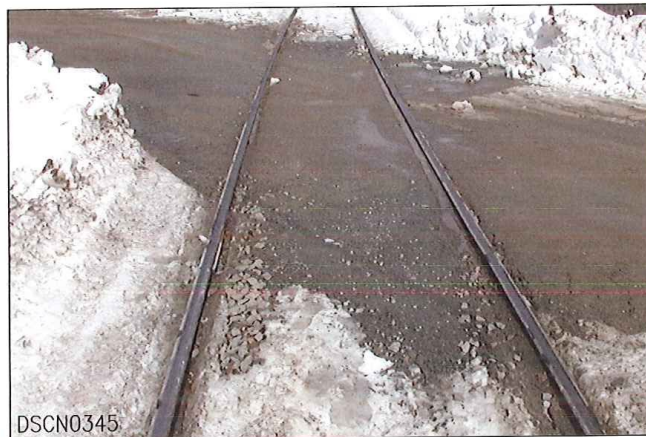
LOOKING FROM WEST TO EAST
