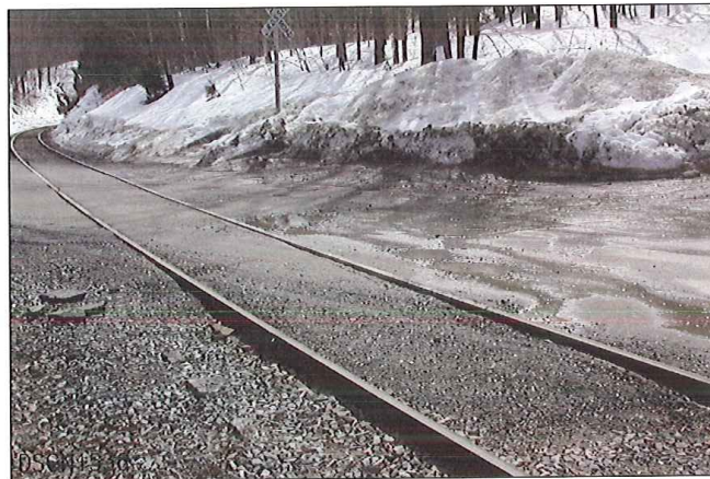
LOOKING FROM WEST TO EAST
