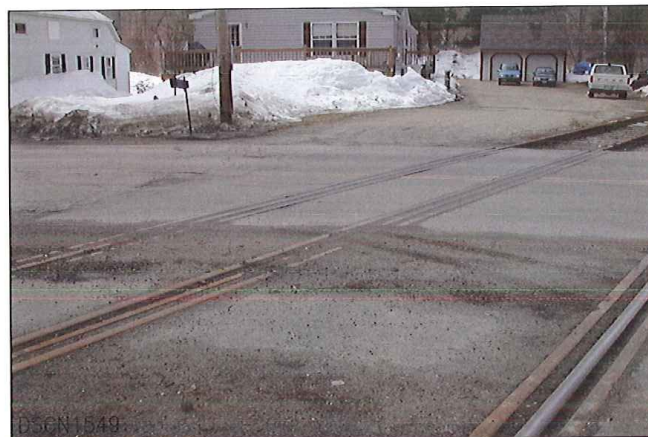
LOOKING FROM EAST TO SIDE TRACK
