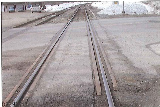
LOOKING FROM EAST TO WEST, MAINLINE
