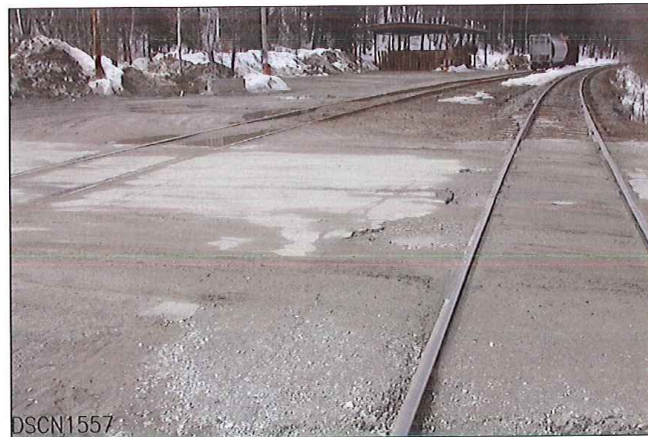
LOOKING FROM EAST TO WEST MAINLINE
