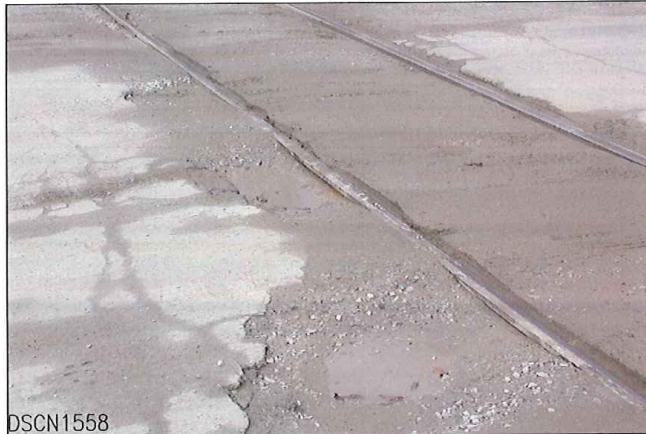
LOOKING AT SOUTH RAIL
