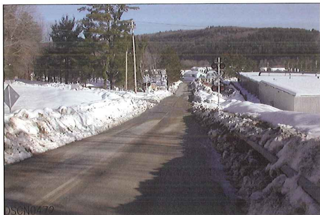
LOOKING FROM SOUTH TO NORTH
