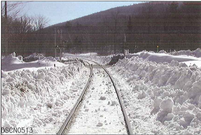
LOOKING FROM WEST TO EAST
