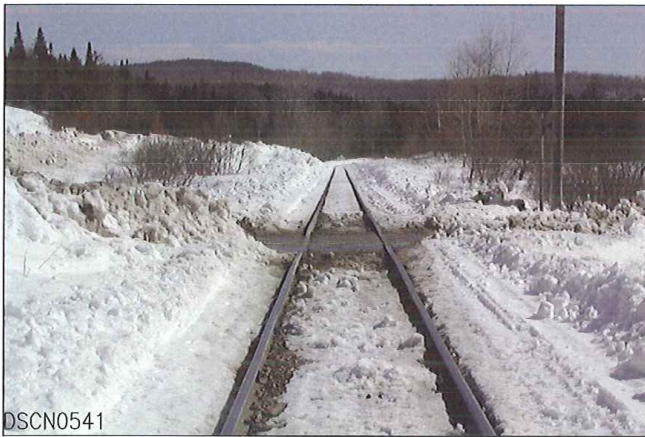
LOOKING FROM WEST TO EAST
