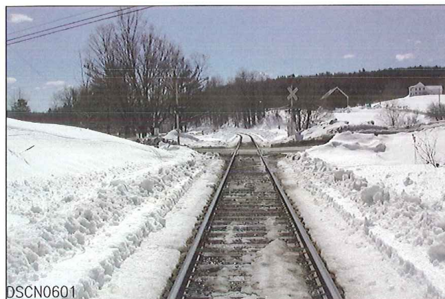
LOOKING FROM WEST TO EAST
