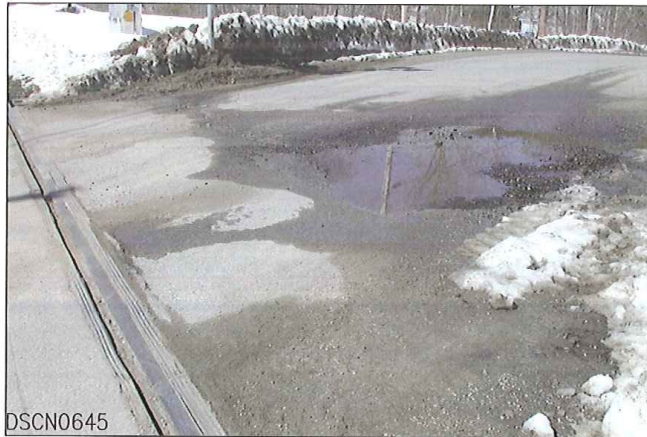
ROADWAY CONDITIONS NORTH OF CROSSING
