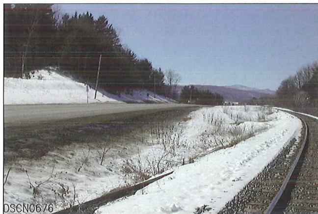
LOOKING FROM WEST TO SOUTH
