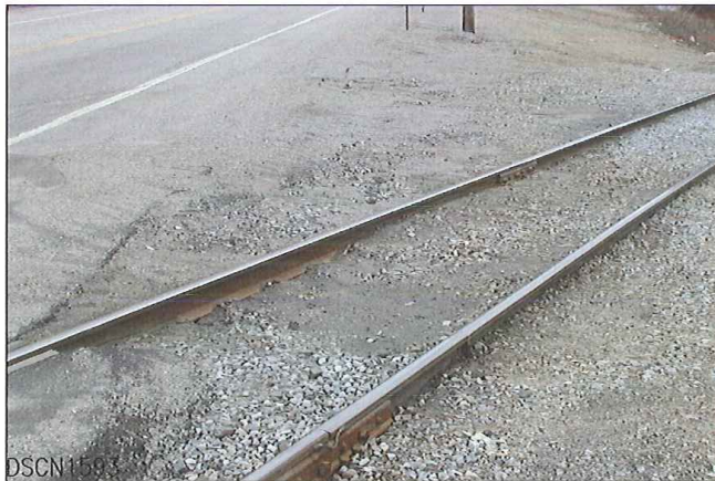
EAST SIDE OF CROSSING
