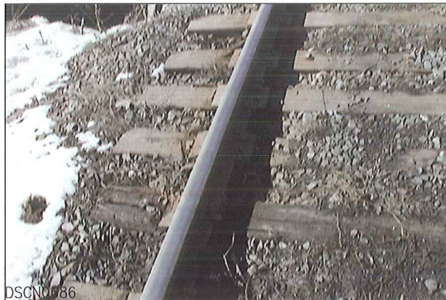
SOUTHEAST QUADRANT AT CULVERT
