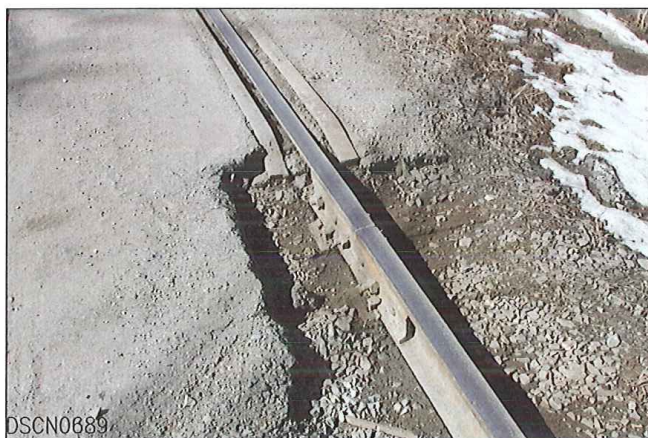
NORTHEAST CORNER OF CROSSING WELD REPAIR
