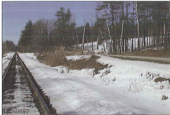
LOOKING FROM WEST TO NORTH
