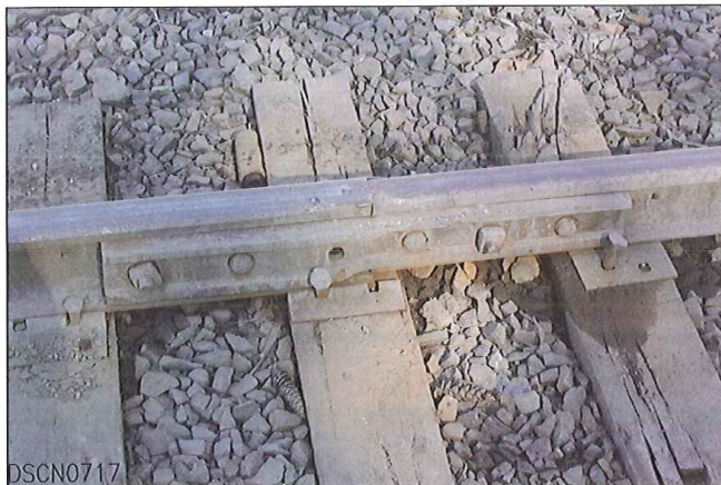
STEP JOINT NORTHEAST RAIL
