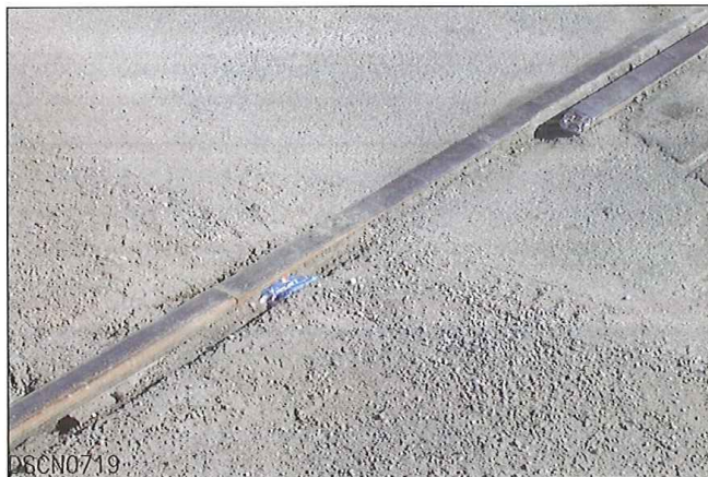
REMOVED NELSON RAIL CHAIR MUDRAIL
