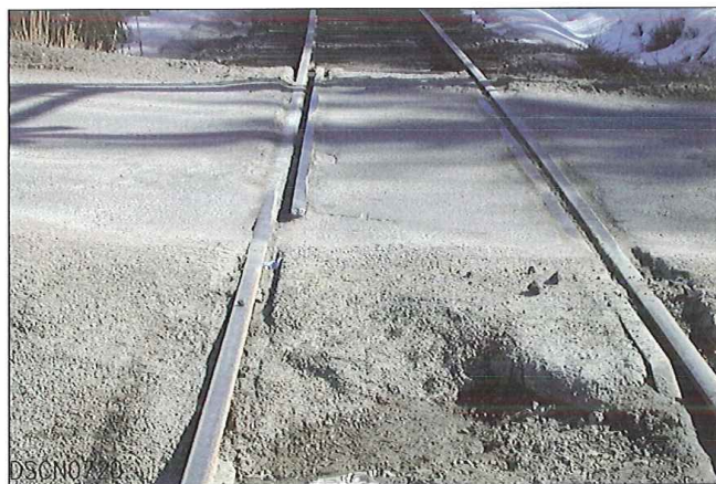
LOOKING FROM WEST TO EAST
