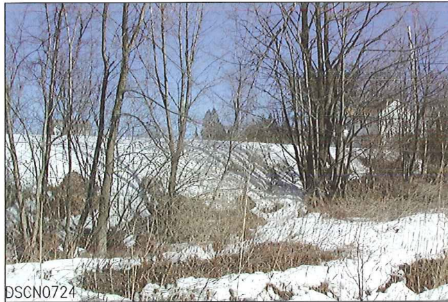
LOOKING FROM WEST TO NORTH
