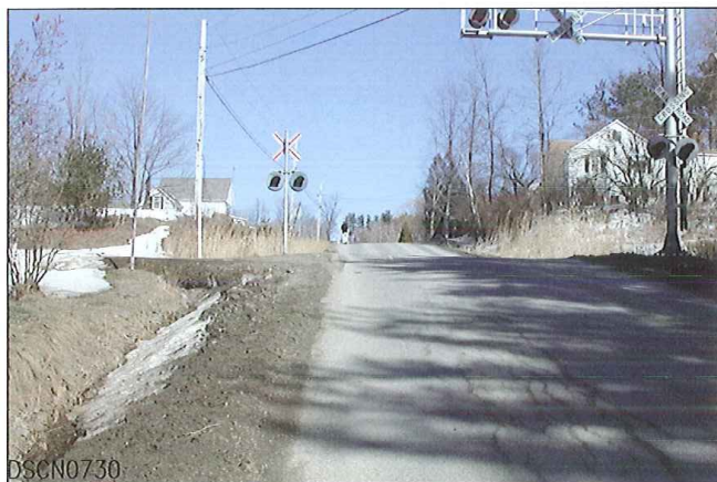
LOOKING FROM SOUTH TO NORTH SUBSTANTIAL UPGRADE
