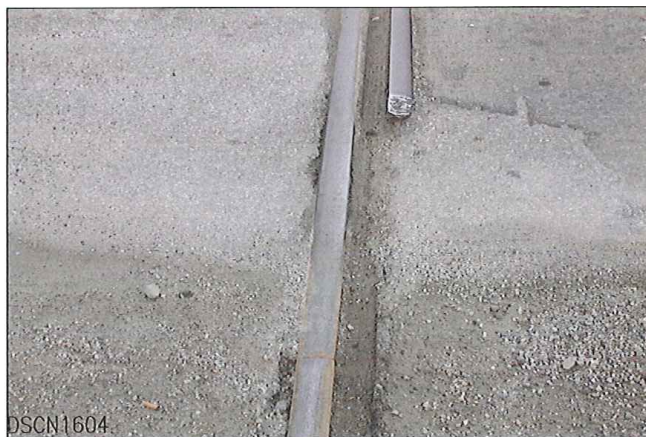
BROKEN MUDRAIL - NORTH RAIL
