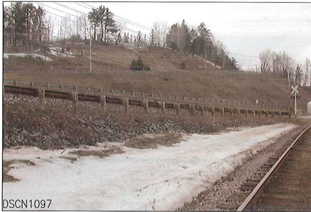
LOOKING FROM SOUTH TO WEST
